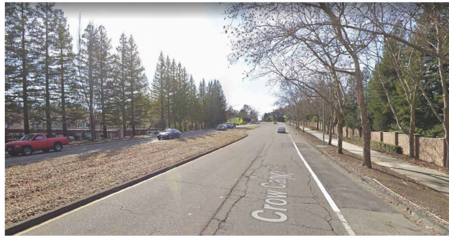
EXISTING CONDITIONS - WEST OF ST GEORGE
